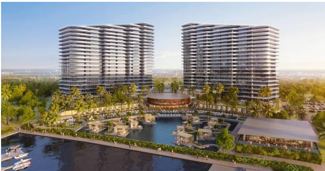
A rendering of the Ritz-Carlton Residences, Estero Bay, in Bonita Springs. Provided by Arquitectonica
