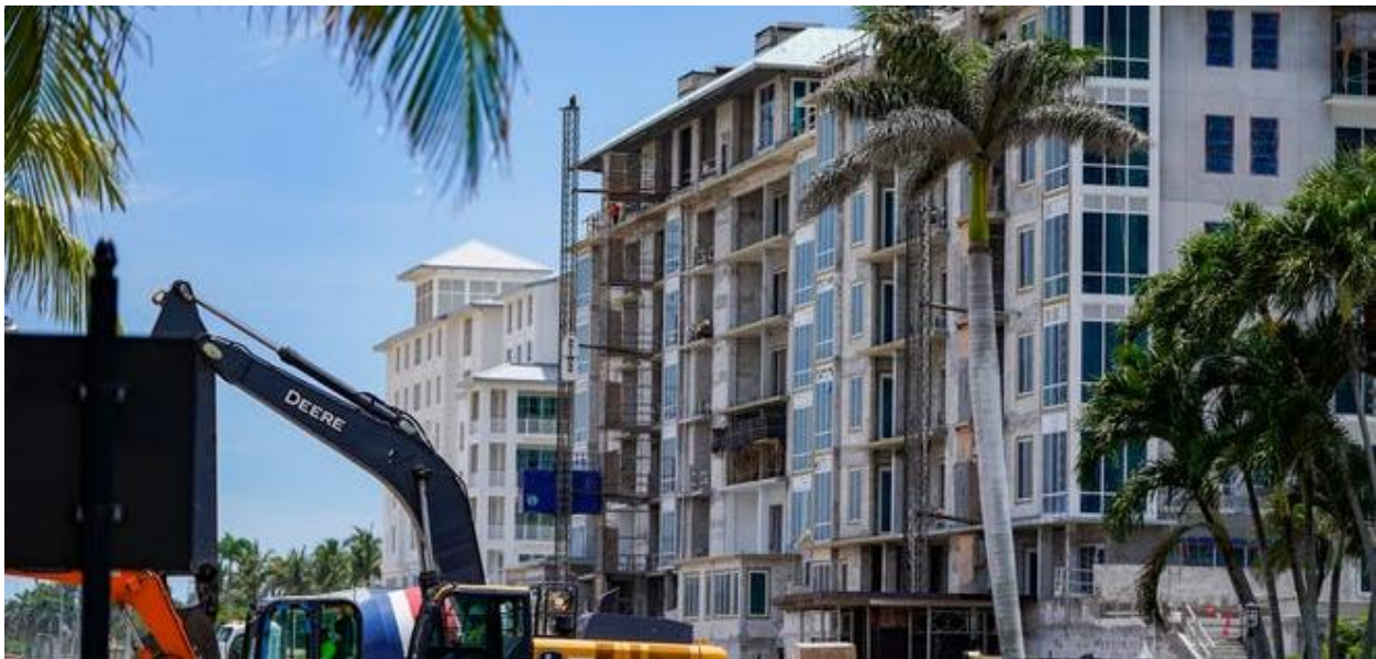
Construction continues at Rosewood Residences and Naples Beach Club
